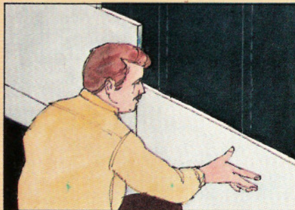
PB2001 AD Protection Panel is applied with AQUASEL PB A2001 AD Protection Panel Adhesive.
